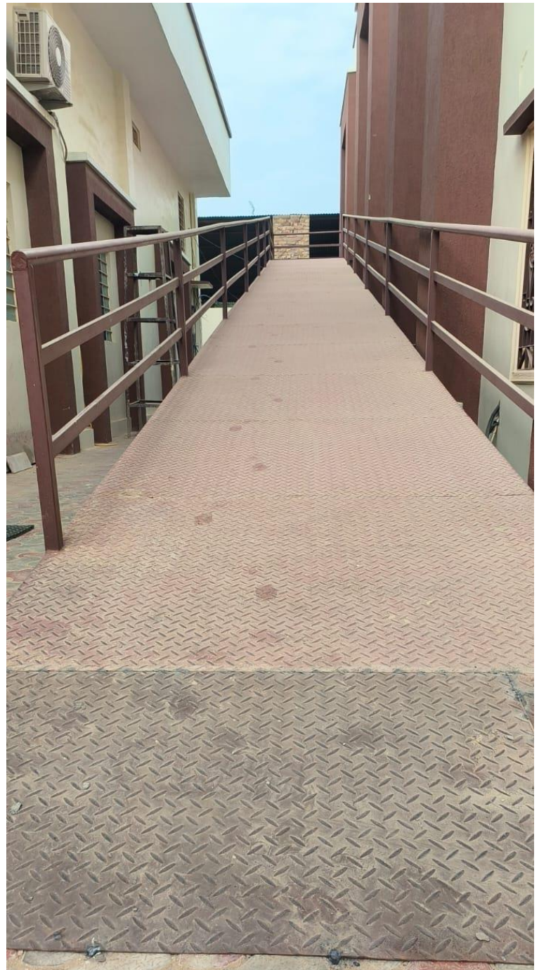
CWSN Ramp to Access First Floor
