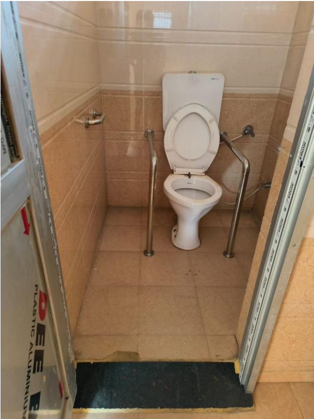
Ground Floor CWSN Toilets for Boys
