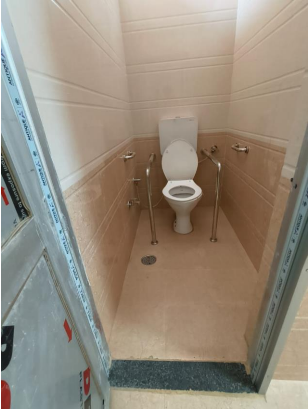
Upper Floor CWSN Toilet for Girls
